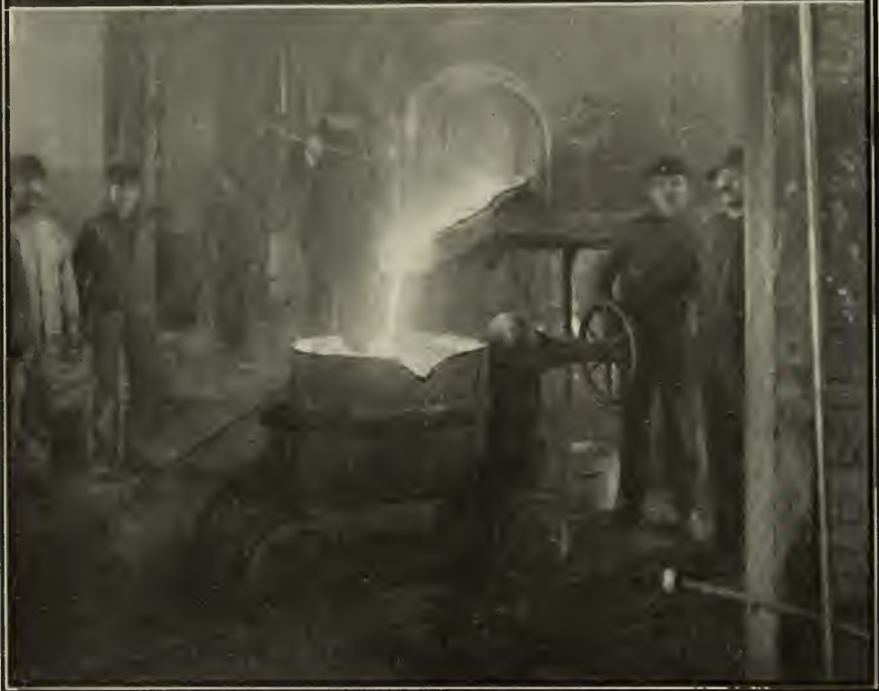
LADLE CAR REVOLVED BY SELF-LOCKING CAM GEAR. FOUNDRY OF THE GENERAL ELECTRIC CO.
